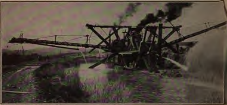
Elevator Dredge Excavating Large Irrigation Canal.
